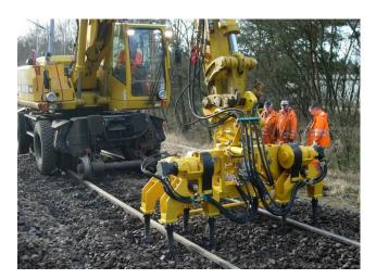
Tamping work at tracks and switches is efficiently executed with the "Attachment Tamping Unit AST 8".
